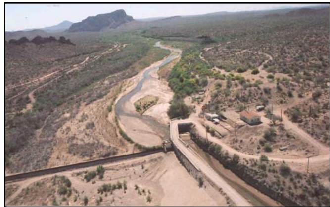
Figure 14. Ashurst-Hayden Diversion Dam, Pinal County, Arizona (Photo by USBR).
